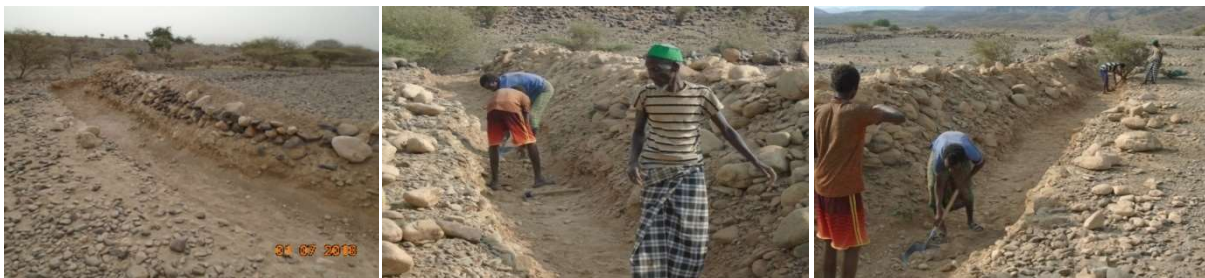
Figure 13 Cut off drain constructed to convey water to its natural course
