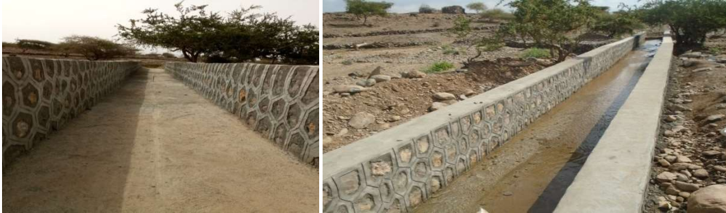
Figure 4: Main canal lining constructed
