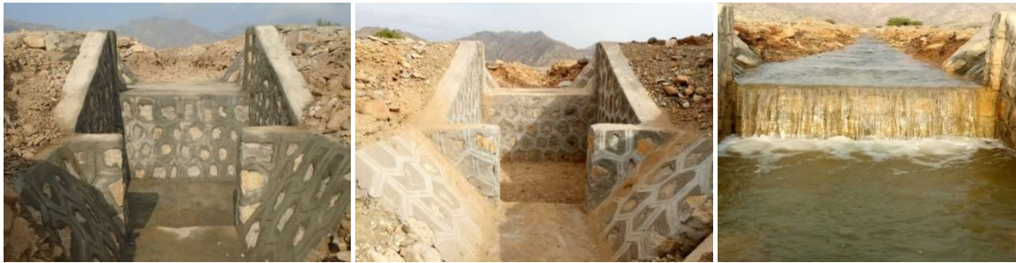
Figure 5: Drop structures constructed on the main canal
