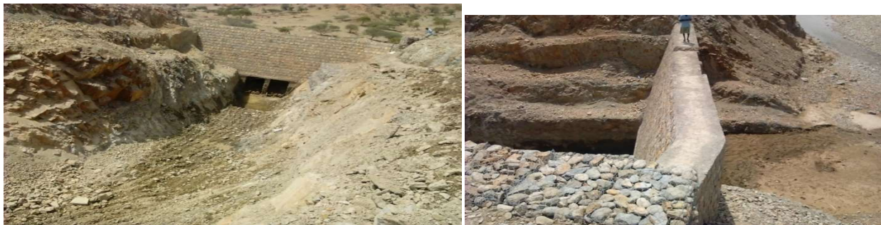
Figure 1 Retaining wall supported with gabion structure
