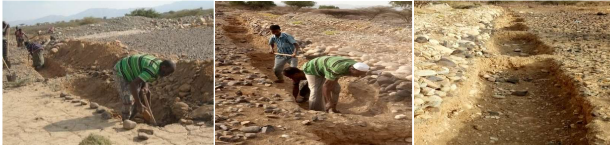
Figure 11 Soil and stone bund constructed
