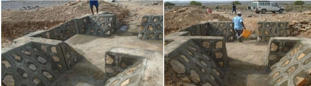
Figure 7: Division boxes constructed
