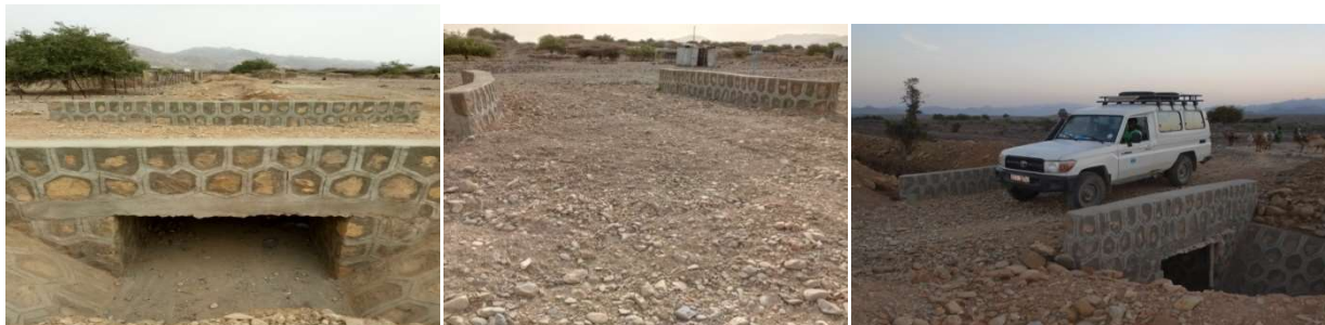
Figure 6: Road and drainage culverts constructed
